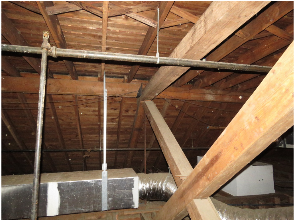
Figure 18: Quarter point rod on east side of Truss 4
