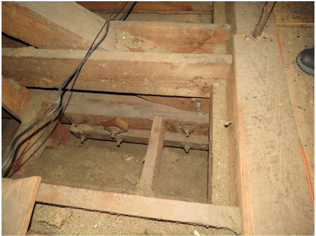
Figure 20: Center rod and bolts at Truss 4 bottom chord
