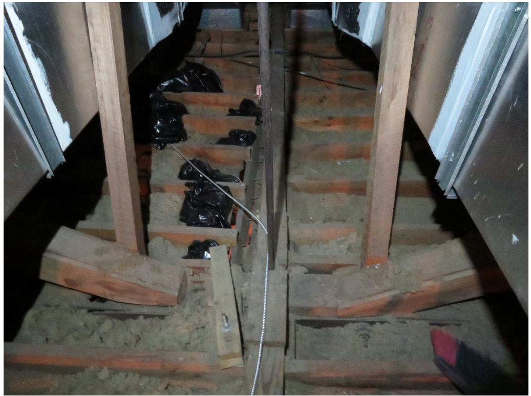
Figure 10: Girder running from Truss 1 to south wall
