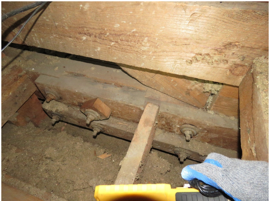
Figure 21: Bolts at Truss 4 bottom chord
