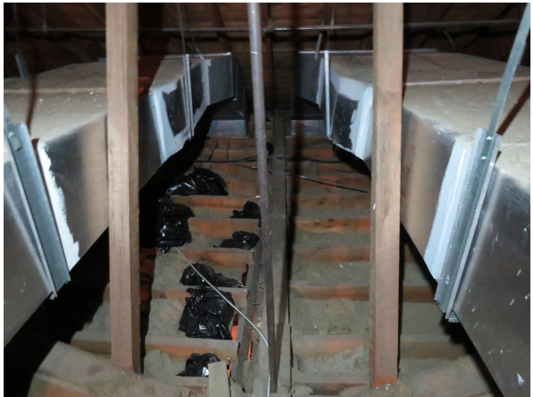
Figure 11: Girder running from Truss 1 to south wall
