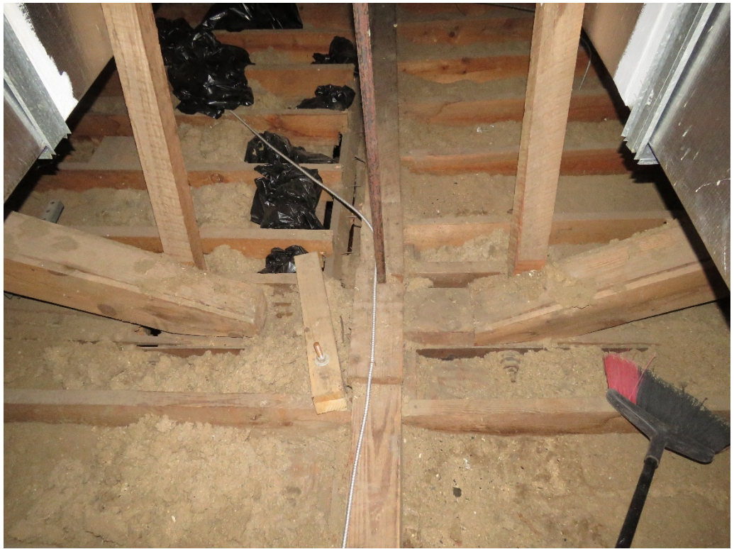
Figure 6: Metal plate side pieces at Truss 1 bottom chord
