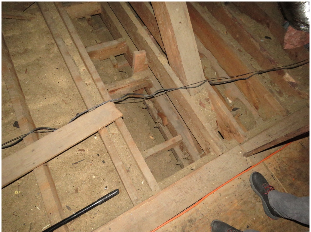
Figure 19: Center rod of Truss 4
